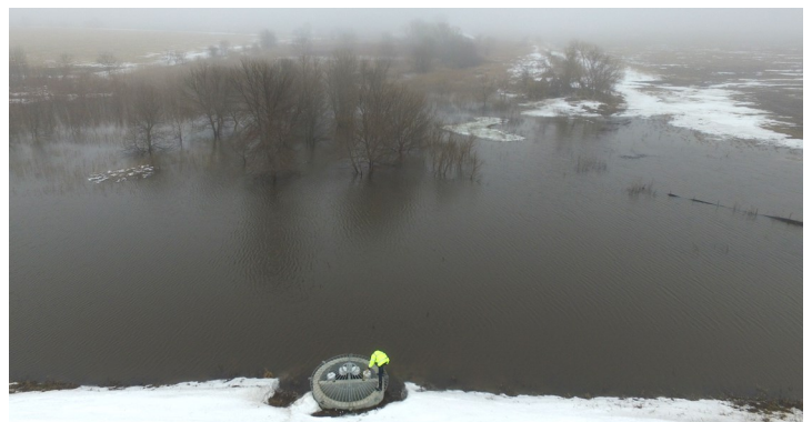
CRWD's Cody Fox checks the flow structure March 9, 2020, at Dobbins 1's upland berm during snowmelt in North Dobbins' headwaters.
